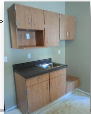
A worker finishing the flooring in the new spa room
