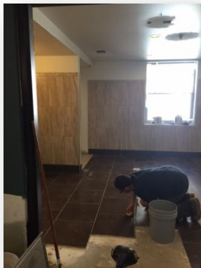
Kitchen area in one of the apartments at Grand Oaks
